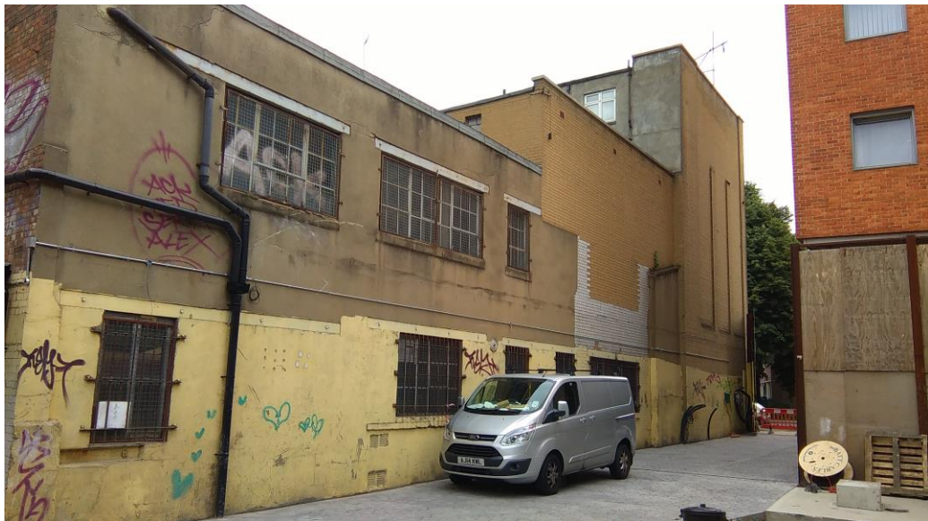
Service yard looking east
