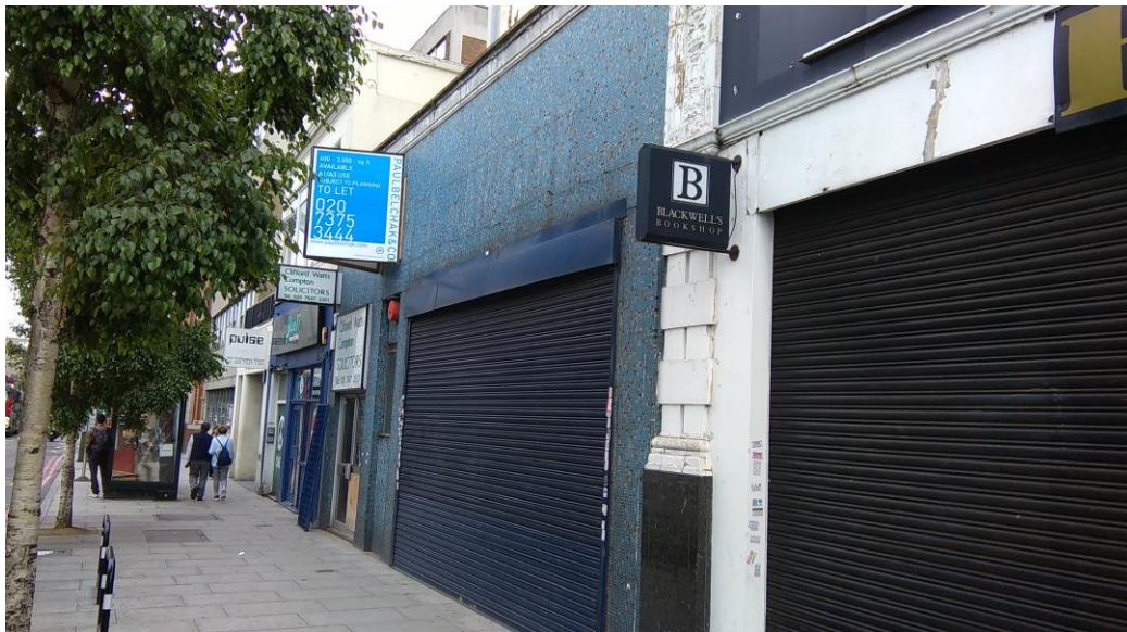
Existing Holloway Road shopfront
