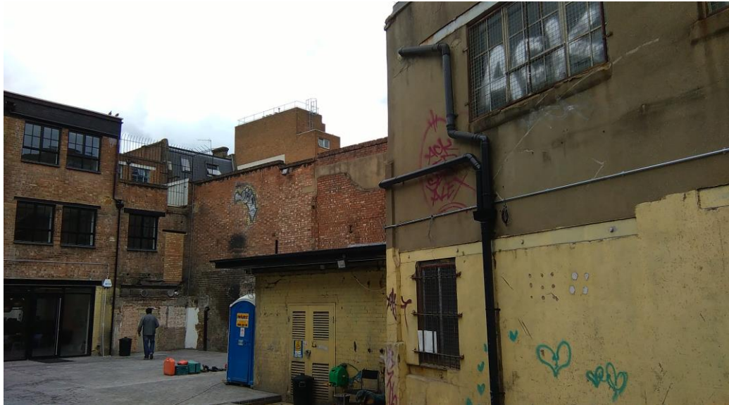
Service Yard looking west
